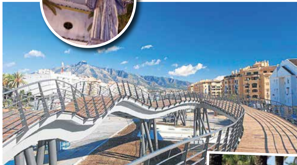
OLD AND NEW: (Above) new bridge and (inset) Iglesia de San Pedro
