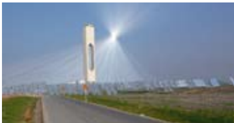
Blazing success - World's largest solar tower near Sevilla
