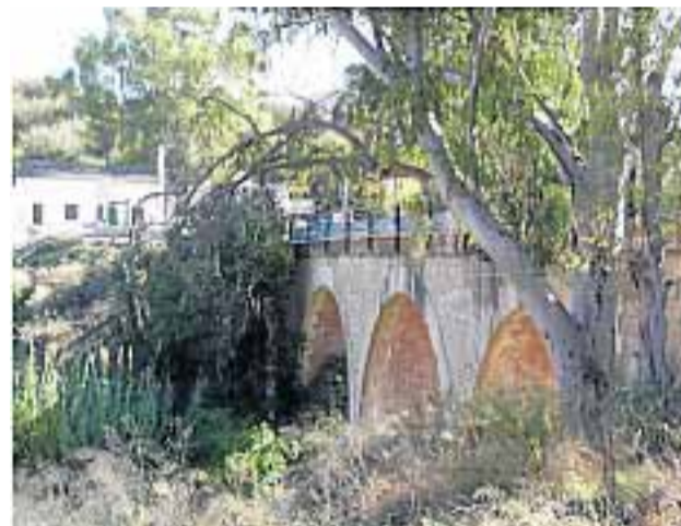
BUILDING BRIDGES: Puente Don Manuel
